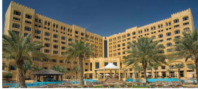
InterContinental Doha Hotel Qatar PARKING SYSTEM
