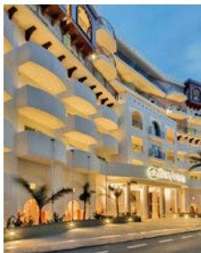
db San Antonio hotel & spa, Saint Paul's Bay Malta PARKING SYSTEMS
