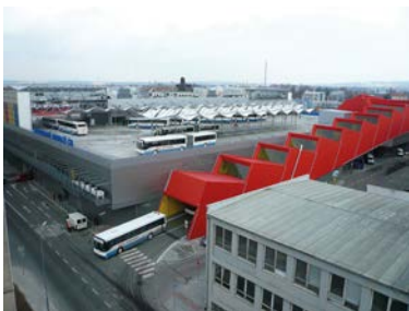
OC Mercury, Ceske Budejovice Czech Republic PARKING SYSTEMS
