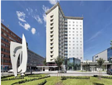
Hotel Continental, Brno Czech Republic PARKING SYSTEM
