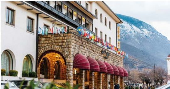
Hotel Dukagjini, Pejë Kosovo PARKING SYSTEM
