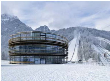
Planica Nordic Centre Slovenia PARKING SYSTEMS
