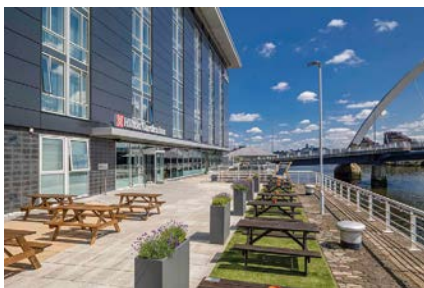
Hilton Garden Inn Glasgow City Centre United Kingdom PARKING SYSTEM
