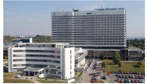
University Hospital Brno Czech republic PARKING SYSTEM
